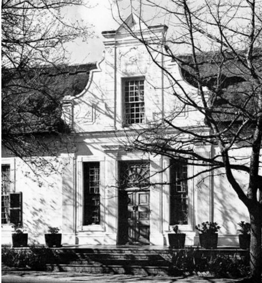
Fig. 6: “La Gratitude”, Stellenbosch, with its thatched roof, pedimental gable and Classical pilasters. Source, Mertens 1971.
