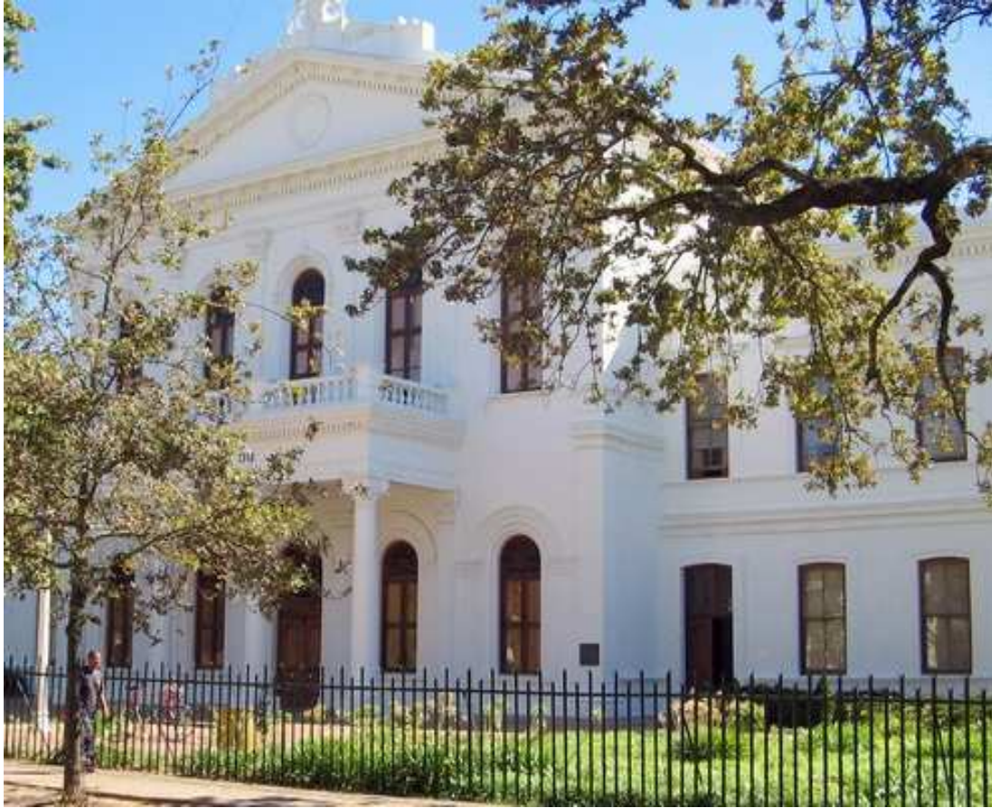
Fig. 3: Old Main Building, Stellenbosch University, 1886.
